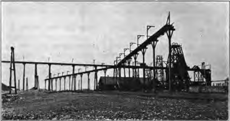
ONE-LEG TRESTLE, COLBY MINE. STOCKPILE CLEANED UP
